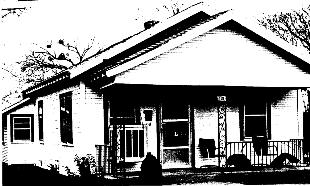
More than 400 homes, like the one above in the JFK project area, have been rehabilitated through the urban renewal program. Photos show before and after effect.
